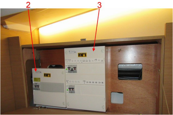
Bipolar circuit breaker (Protection) Ref 2
